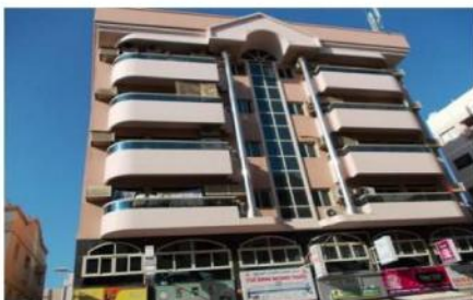
AMAF Bin Sanquor Building
